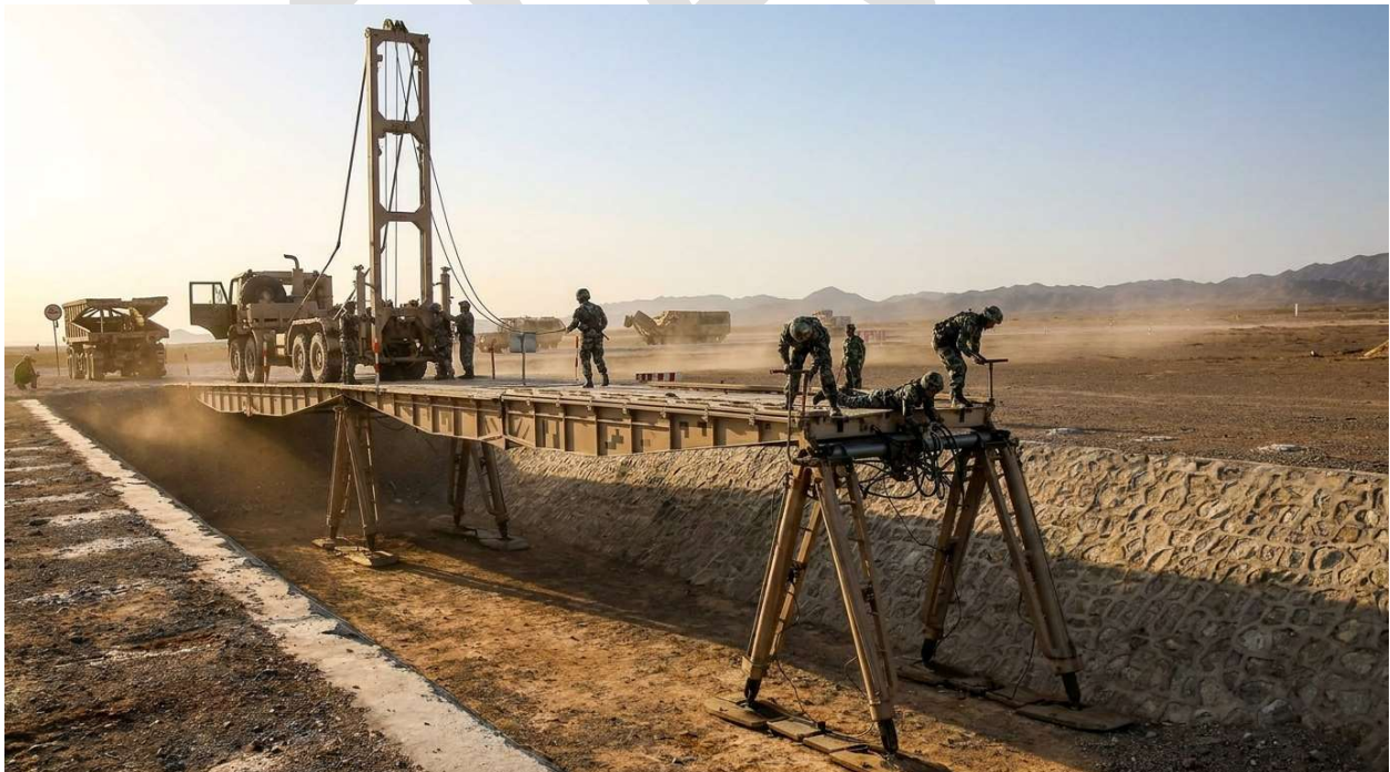
Figure 5.13 – GQL-111 bridge laying across a dry gap demonstration
