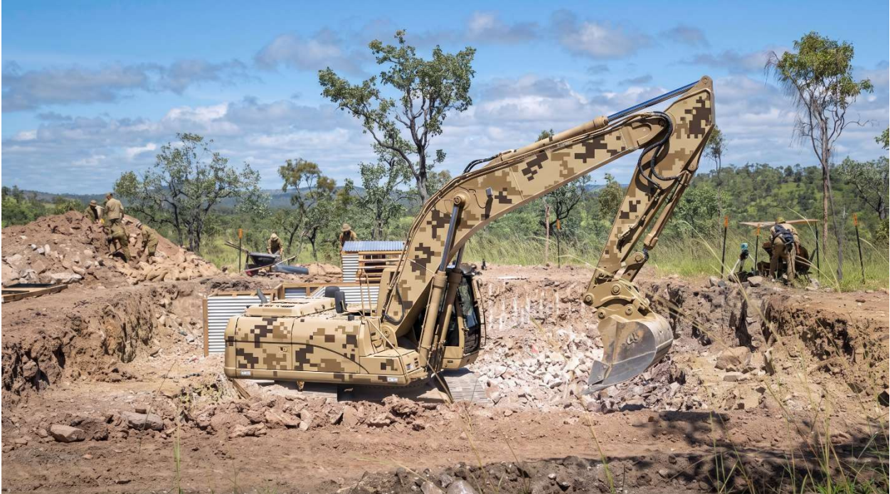
Figure 8.1 Preparatory excavation works using plant
