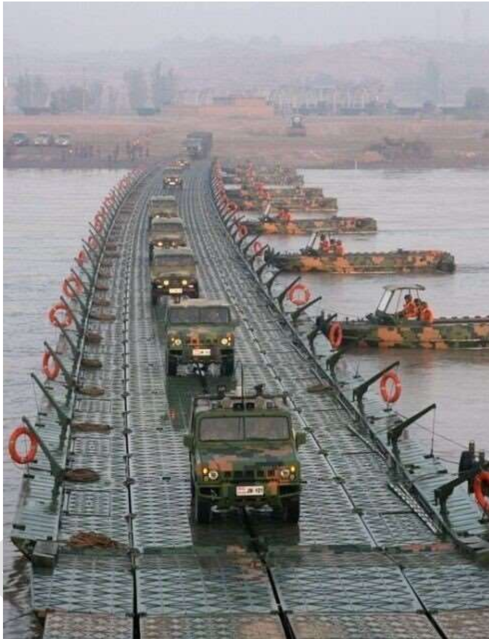
Figure 5.15 Completed Ribbon Bridge
