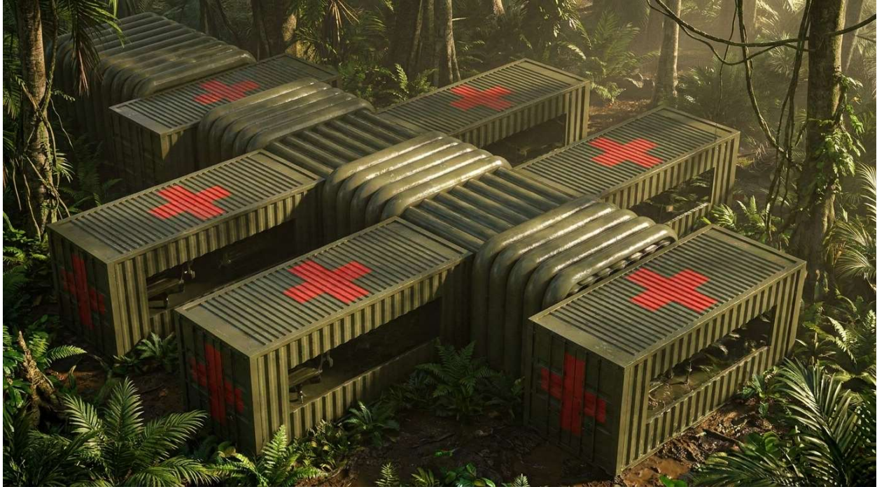
Figure 8.2 Surface laid ISO container based hospital
