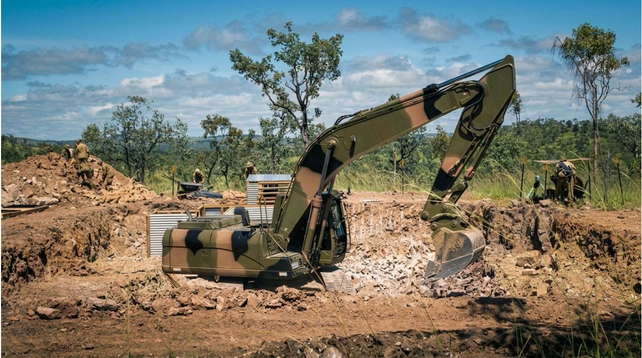
Figure 8.1 Preparatory excavation works using plant
