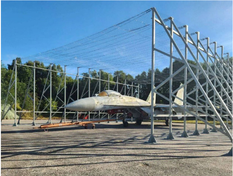
Figure 7.7: Experimental Russian anti-drone screen. Basic construction of frame, wire and mesh screen
