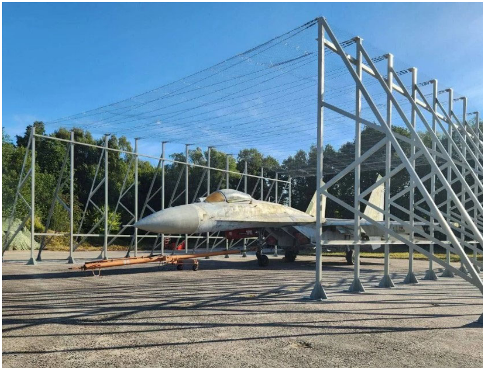
Figure 7.7: Experimental Russian anti-drone screen. Basic construction of frame, wire and mesh screen
